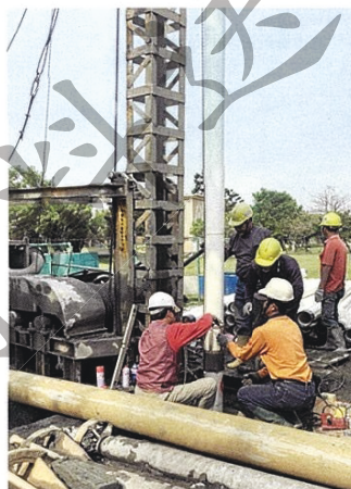
鑿井工程 Well drilling engineering
